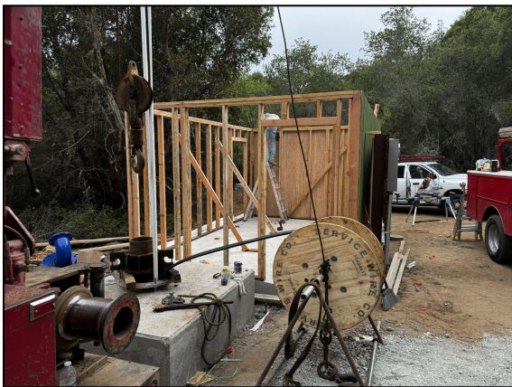
Construction of the Pump Station Building
