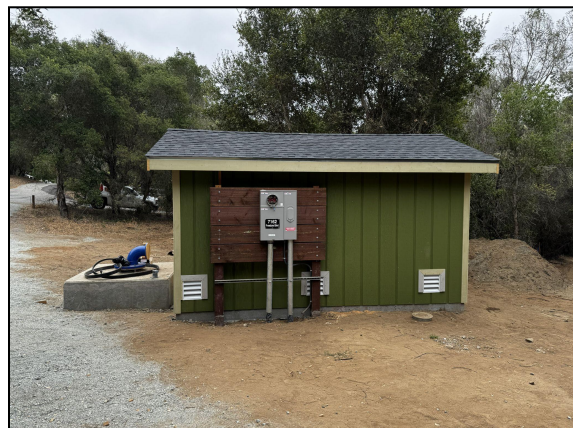
Pump Station Building Completion
