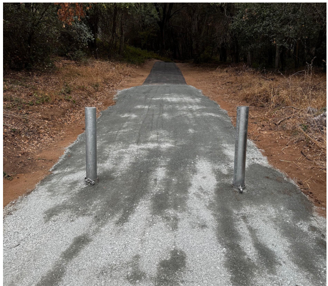
Access Road with bollards.
