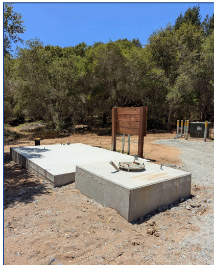
Well 14 foundation for Pump Station building.
