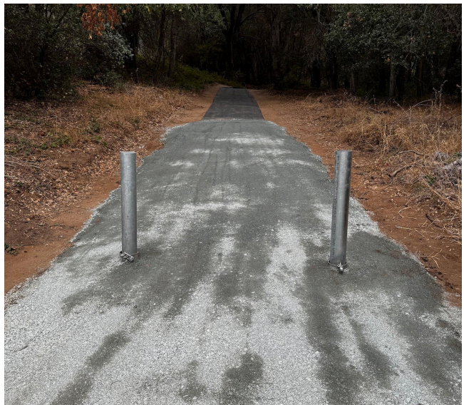
Access Road with bollards.
