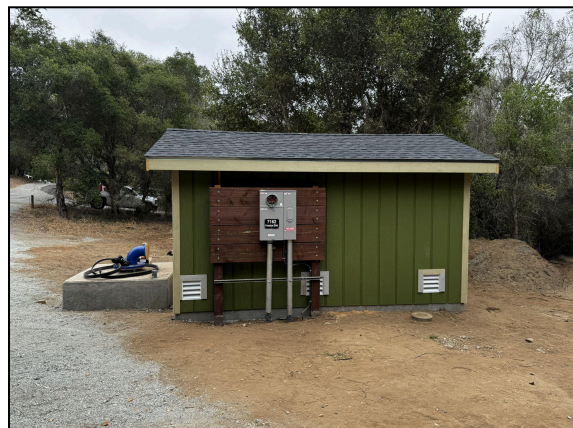
Pump Station Building Completion
