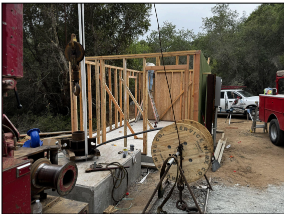
Construction of the Pump Station Building
